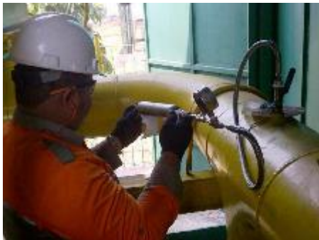
Gas heating value is verified with direct gas sampling
